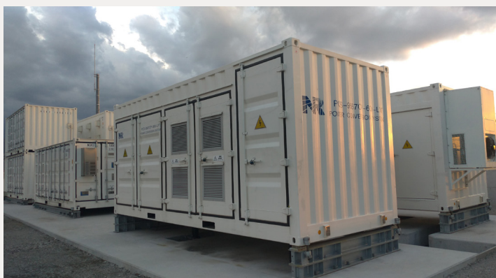
1.2MW/7.2MWh NGK Shikoku Island ITO sodium-sulfur battery energy storage project, Japan
