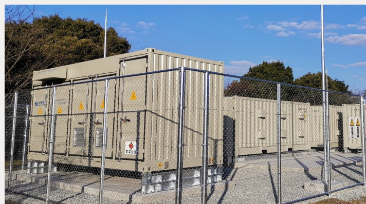
600kW/3.6MWh TOTO factory user-side sodium-sulfur battery energy storage project, Japan
